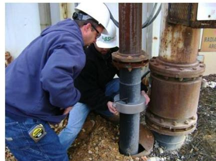
Figure 2. Installation of original array/cover on a vertical slurry line adjacent to a flange.
