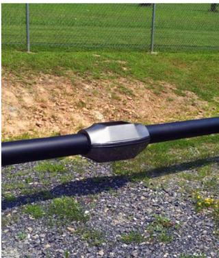
Figure 1. Ultrasound array with solar collector integrated into housing.
